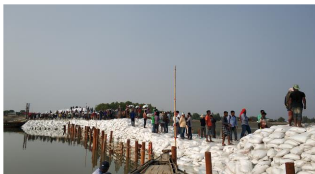
Figure 3-11: Nalian Closure Dam of Polder-32 (completed)
