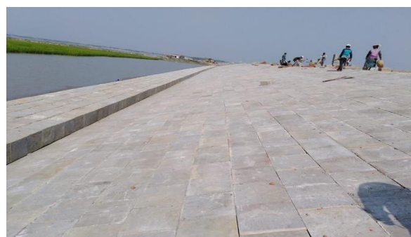
Figure 3-10: Completed Slope Protection Works in Polder-32
