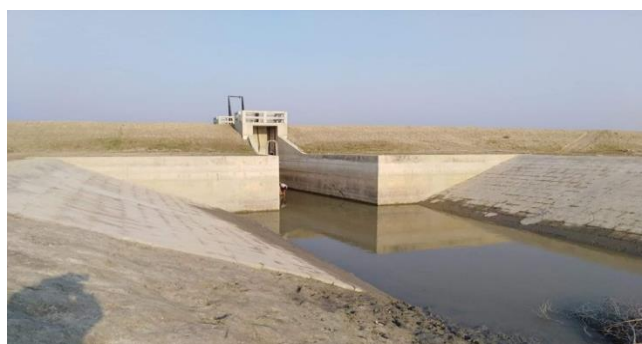
Figure 3-9: Completed DS of Polder-32
