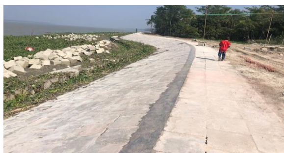
Figure 3-26: Bank Protection with Pitching Works (Polder 39/2C)
