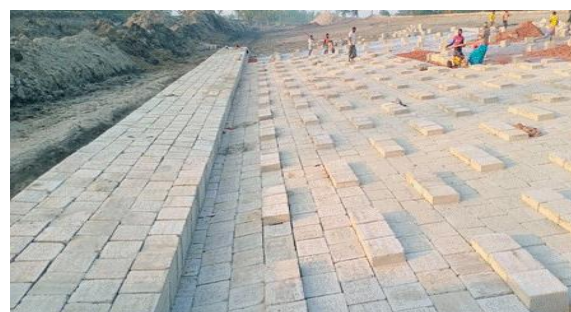
Figure 3-27: Ongoing Slope Protection Works (Polder 40/2), Barguna
