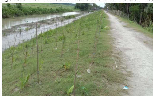
Figure 3-31: Grassing from k9+600 to k10+700 in Polder-43/2C
